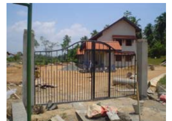
Main gate under construction
